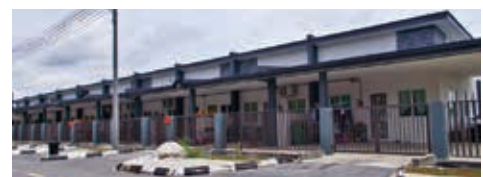
Single-Storey Terrace House. Intermediate Unit, Standard Lot Size: 18 Feet x 65.6 feet. Built up area: 632 square feet.
